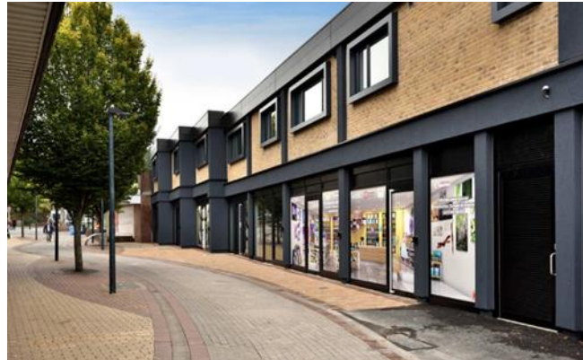
Limes Walk, Oakengates
