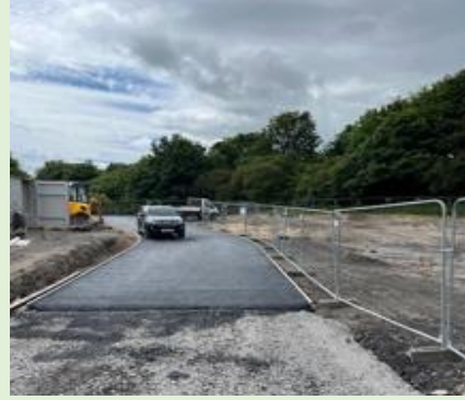
Pool Hill Road Site D – in progress
