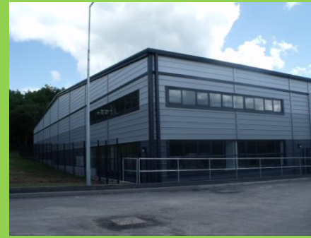
T54 – Plot 5c TWC industrial unit – Operational – Filtermist
