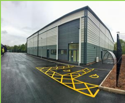
T54 – Plot 5a TWC industrial unit – Operational – Incomm Training
