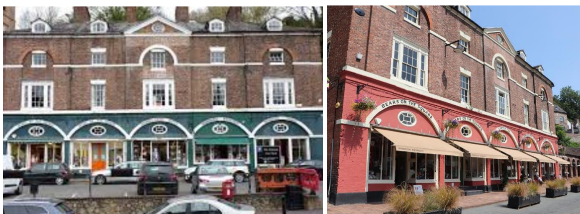
Shops in the Square, Ironbridge Before & After Façade Improvements
