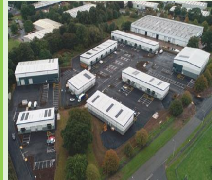
Hortonwood Plot 12 – TWC – Operational
